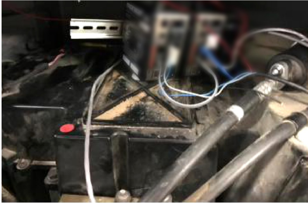
Figure 2: Field-deployed telematics instrumentation in a protected equipment compartment. Continuous capture of engine-control parameters at engine-cycle cadence supports the diagnostic substrate; the same physical install supports both the diagnostic-event use case and the continuous-monitoring use case described in Section 4. (2018 field deployment context.)
